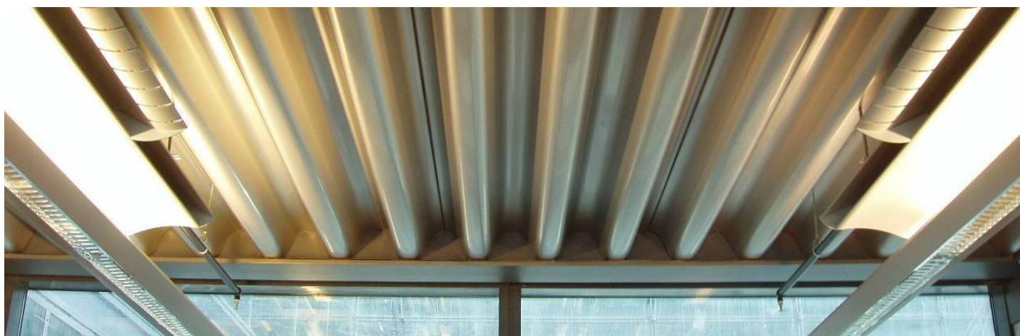
Figure 1: Profiled stainless steel decking
